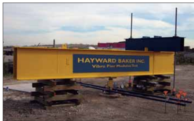
Vibro Pier Modulus Test to verify system performance.
